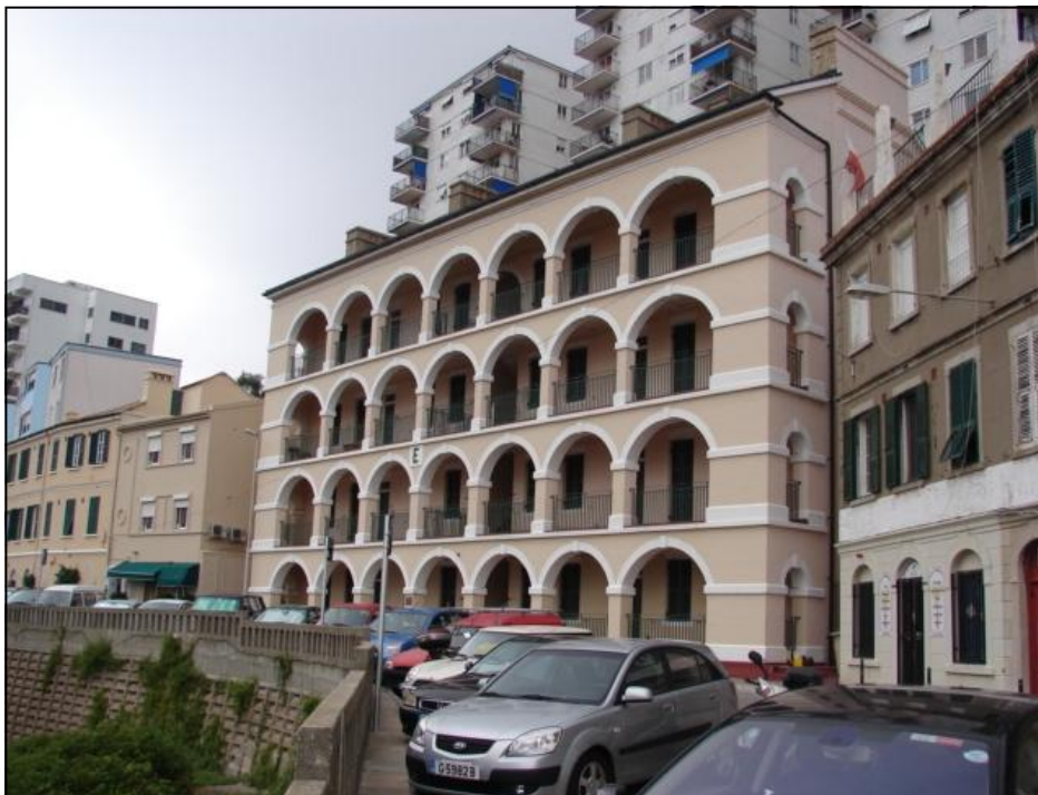
Eight two bedroom apartments situated at Naval Hospital Road.
